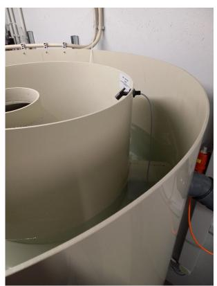
The ClearFox® DAF is a fully automated unit. The wastewater to be treated is fed from the customer's surge tanks or the ClearFox® buffer tanks of the DAF via a non-clogging cavity pump. The use of aerated buffers is recommended for certain applications.
